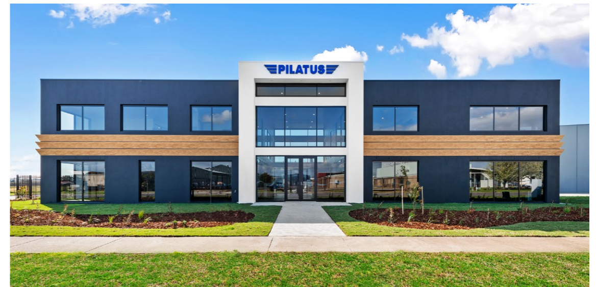
The new headquarters of Pilatus Training Solutions Australia Pty Ltd in Sale, Australia
